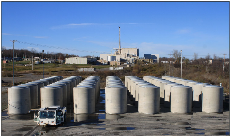
High-Level Waste from the West Valley Demonstration Project in Interim On-Site Storage, March 2017
