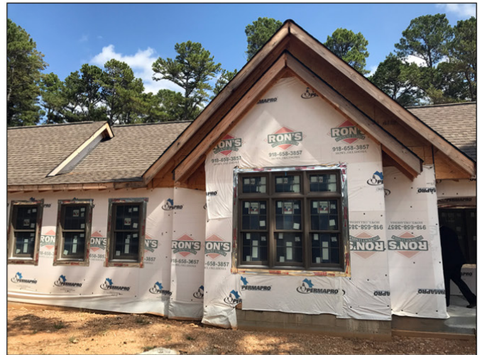
Choctaw Nation Multiroom House Under Construction
