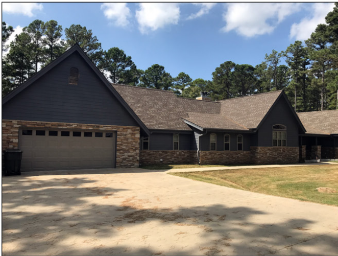
Choctaw Nation Completed Multiroom House
