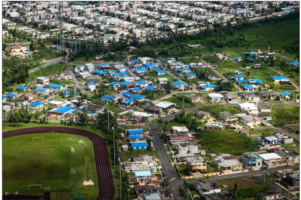
Figure 7: Temporary Blue Roofs in Puerto Rico Installed by the U.S. Army Corps of Engineers after Hurricane Maria in February 2018
