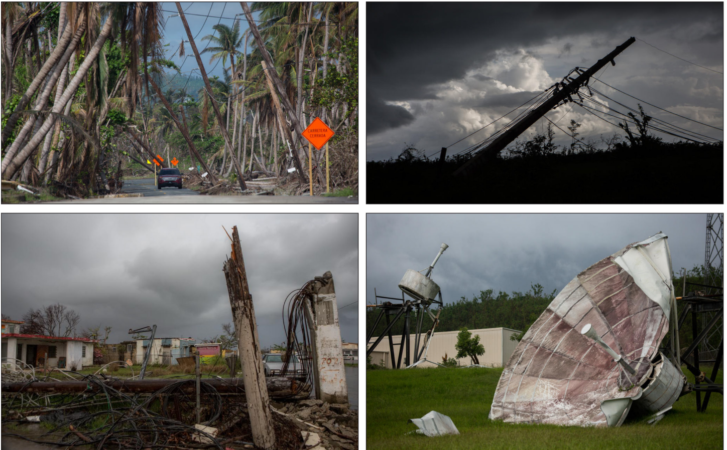
Figure 10: Damaged Power Lines and Satellite Dish in Puerto Rico after Hurricane Maria in November 2017
