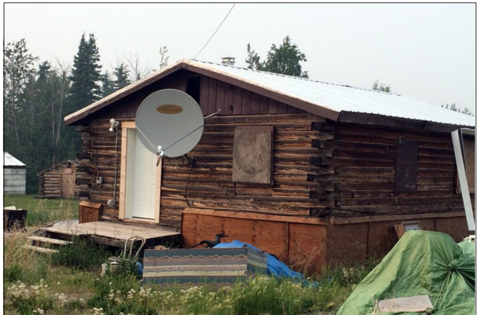
Figure 3: A Building in Beaver, Alaska Serviced with a Satellite Internet Connection
