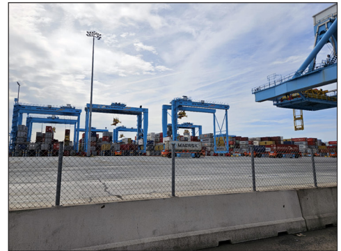
The automated area of the terminal (the yard) is fenced off from areas with workers, reducing the potential for injuries.
