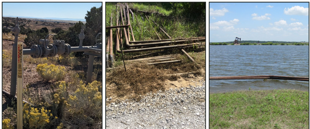
Figure 2: Examples of Gathering Lines and Associated Infrastructure
