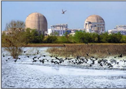
South Texas Project, reactor units 1 and 2
