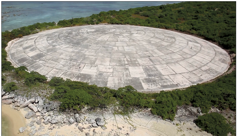
Figure 17: Runit Dome after Construction in 1979 on Runit Island, Enewetak Atoll
