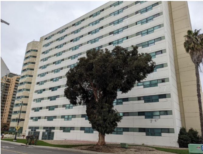
A 12-story barracks without air conditioning
