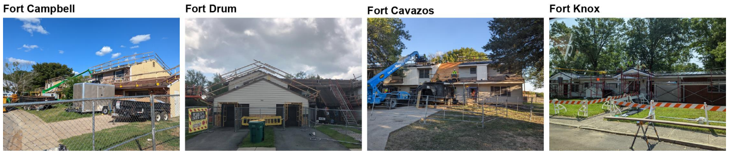
Figure 12: Examples of Integrated Development Plan Roof Replacements
