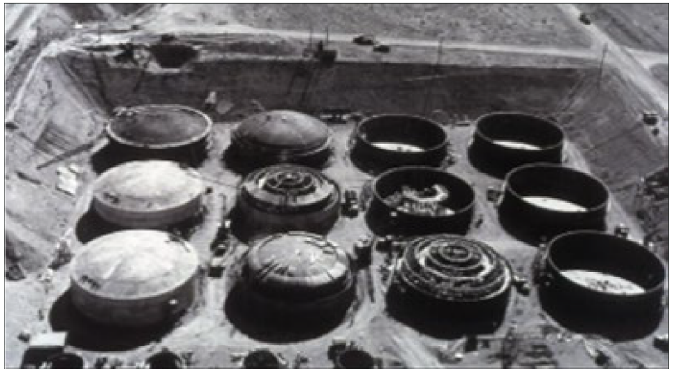
Figure 1: Hanford Single-Shell Tank Farm under Construction
