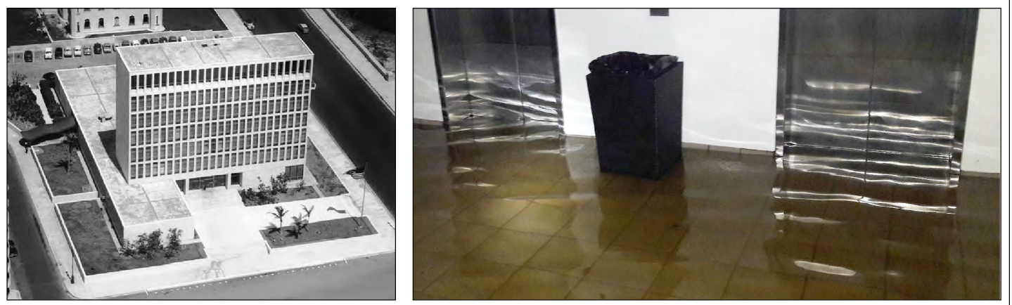
Figure 1: U.S. Embassy Havana, Cuba as Built in the 1950s (left), and Flooding within the Elevator Lobby from Hurricane Irma in 2017 (right)
