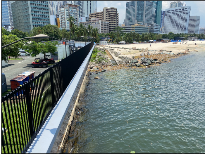
Manila Bay sea wall and stormwater outlet.
