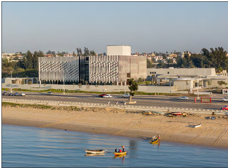
Exterior facade to reduce building heat gain.
