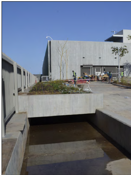
Storm water retention basins.
