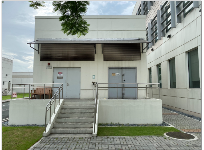
Chancery generators relocated and elevated.
