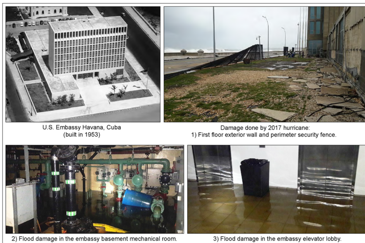
Figure 1: Damage to U.S. Embassy Havana, Cuba from Hurricane Irma in 2017
