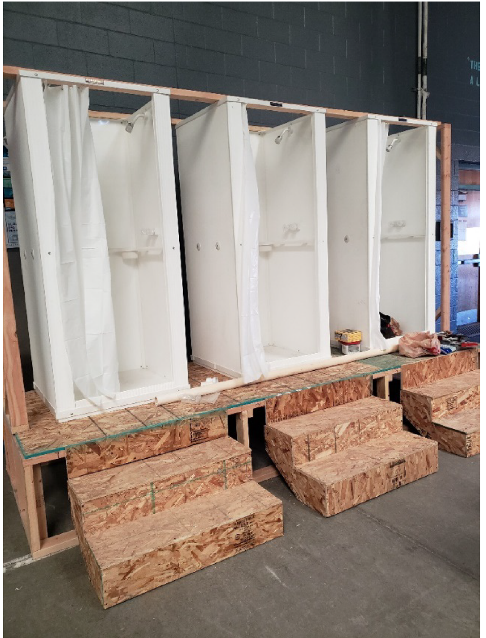
Figure 14: A Federal Bureau of Prisons Facility's Installation of Temporary Showers in Alternate Housing Areas for Inmates in Quarantine and Isolation
