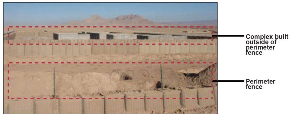
Figure 1: Compound Comprising Five Buildings Constructed in a Non-secure Location outside the Perimeter of a Base
