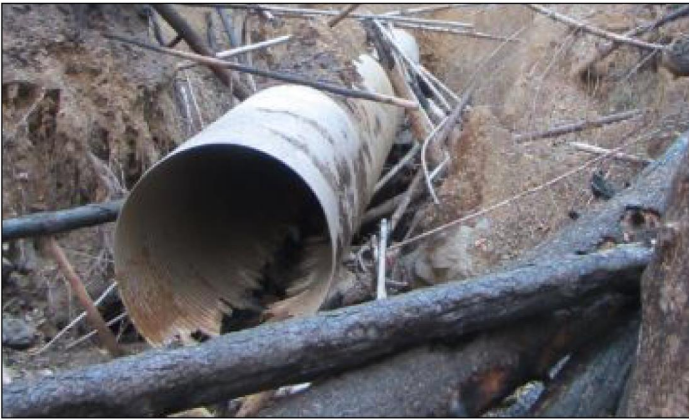
Figure 9: Culvert and Road Damaged by Erosion following the Chetco Bar Fire, October 2017
