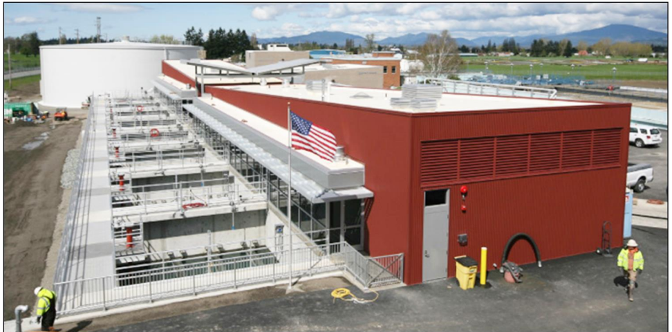
Figure 4: New Waterproof Drinking Water Treatment Plant, City of Anacortes Public Works
