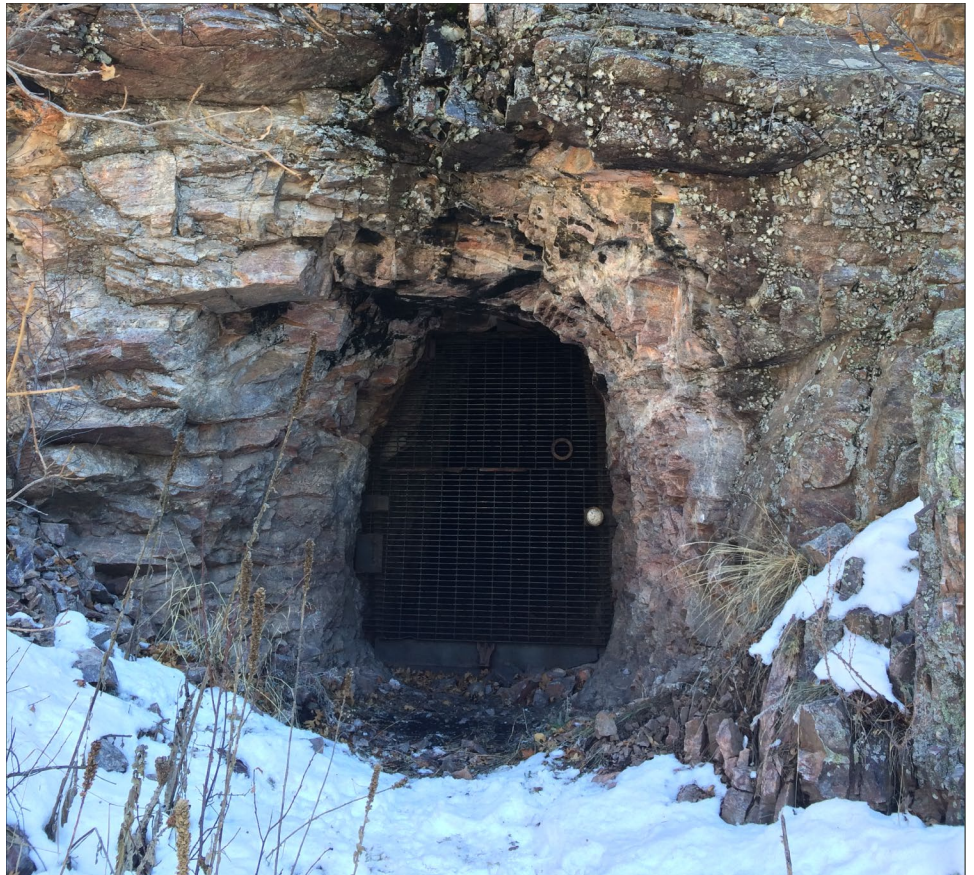
Figure 4: Abandoned Hardrock Mine Tunnel Opening Secured with a Gate to Allow Bat Access on Bureau of Land Management Land in Colorado
