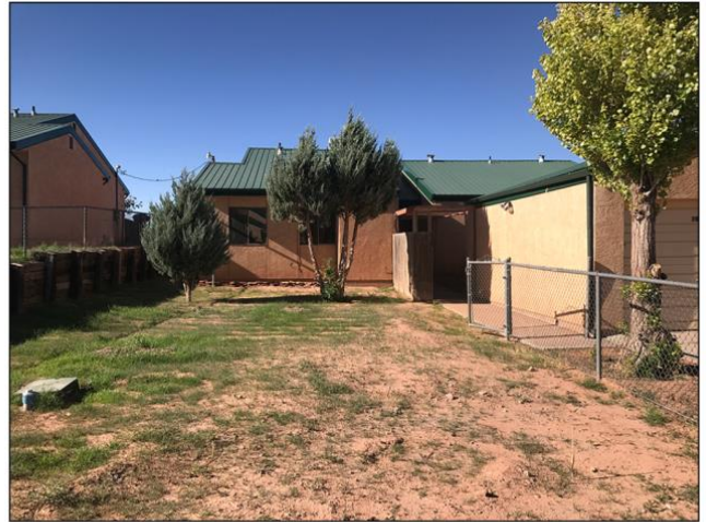
Chinle Comprehensive Health Care Facility
