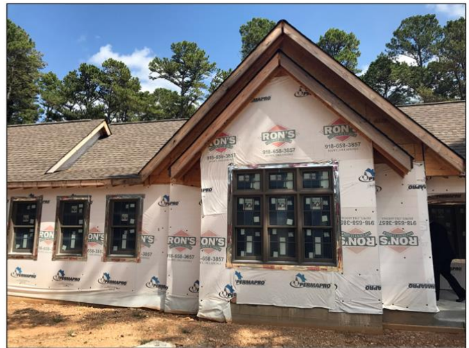
Choctaw Nation Multiroom House Under Construction
