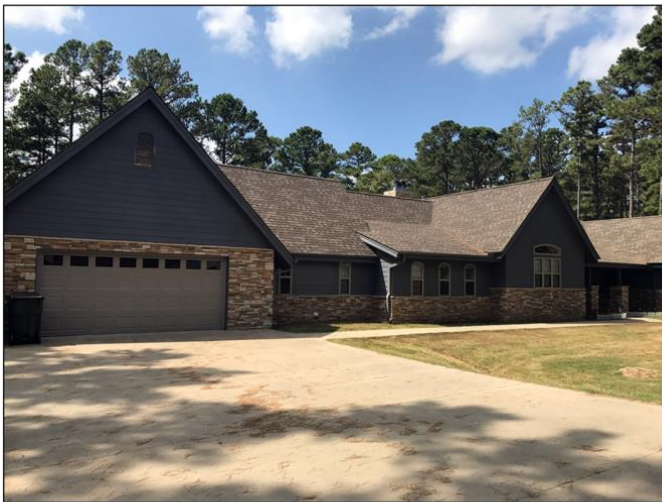
Choctaw Nation Completed Multiroom House
