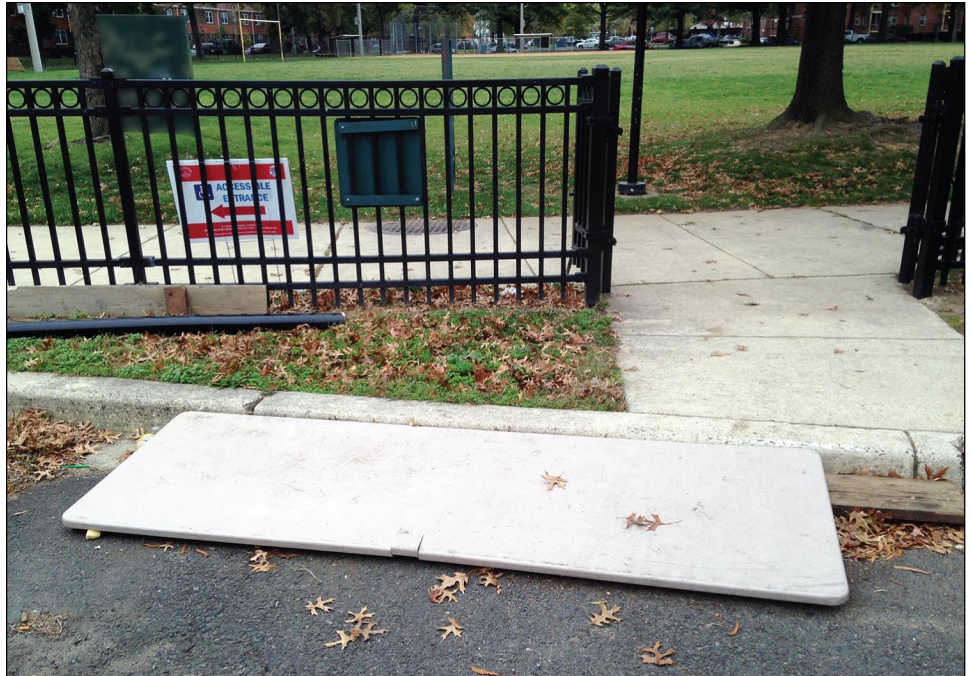
Figure 6: Example of a Polling Place with a Make-shift Ramp Constructed from a Folding Table and a Block of Wood That Could Pose an Impediment for Voters with Disabilities
