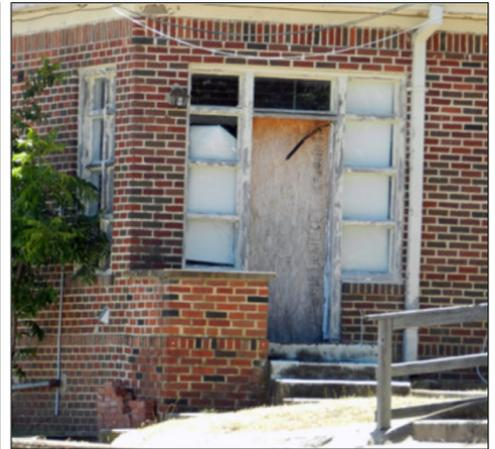
Exterior view of the building shows broken windows, and missing bricks.
